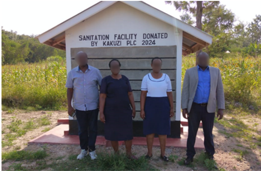
Photos 4: Handing over of 4 -door ablution blocks at Mwanja Mbogo dispensary
