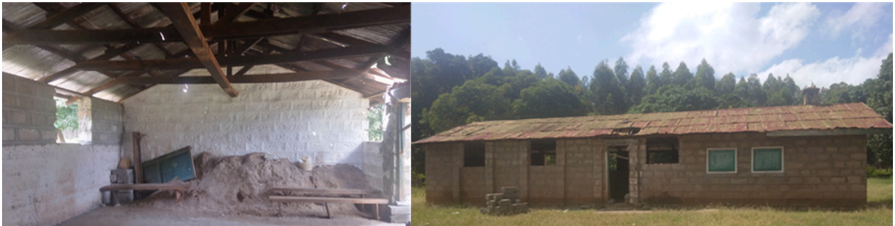
Photos 14: Kabatini forestry hall under renovations
