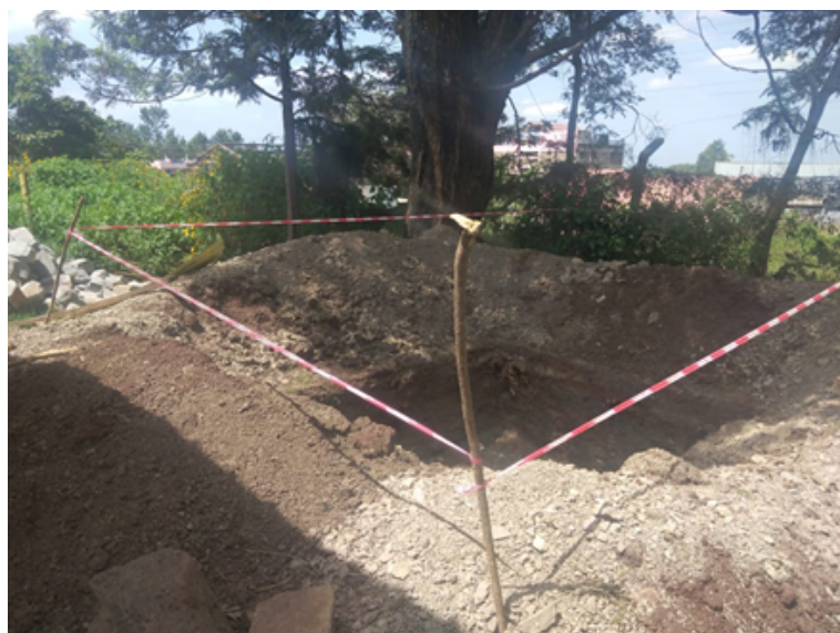
Photos 10: Ongoing Construction of a 4- door sanitation facility
