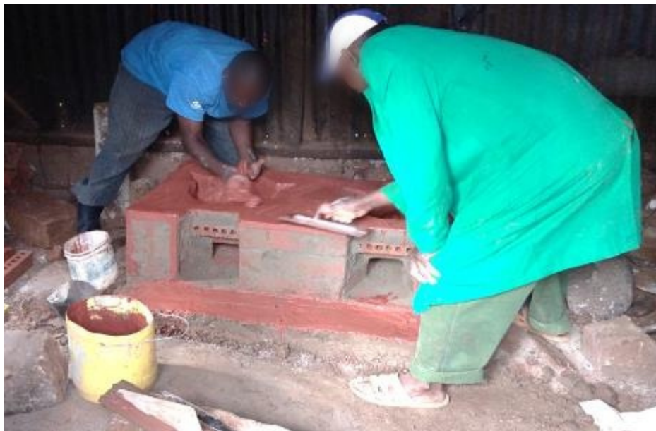
Photo 7: Builders during Installation of energy saving jiko (jiko kisasa)
