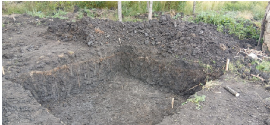
Photos 8: Construction of 4 door latrine at Mangoto Primary School
